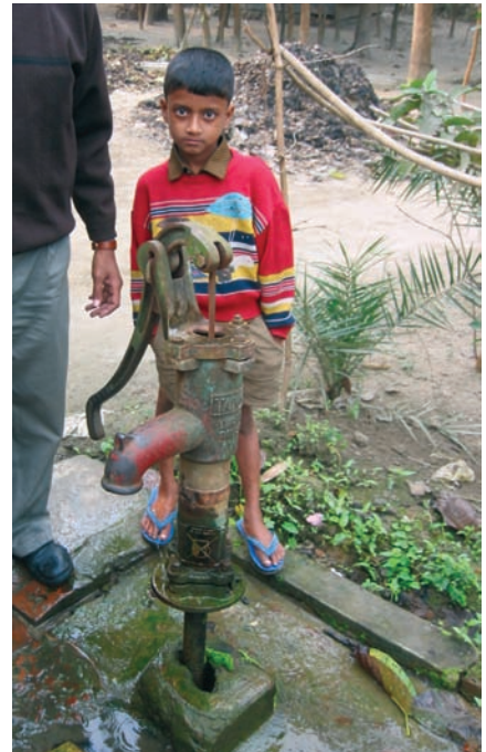
PLATE 4. Resources for drinking water. Upper left: Guanxi, China (2006). Dug well with hand pump. Cement cover to protect the water. Upper right: Rural Malaysia (1974). High school lesson for making a safe well: Common dipper, so individual pails don't contaminate; protected by fence, so chickens, other animals, and small children don't fall in. But really useless, with water table so high and contaminated water so near. Lower left: Rural Punjab, India (1984). Residential tube well in Punjab as Green Revolution prosperity transformed water safety. Lower right: Rural Bangladesh (2007). Shallow tube well painted red because of high arsenic concentrations. Arsenic occurs naturally in the shallow aquifer in much of rural Bangladesh and causes cancer when water from these wells is drunk over long periods.
